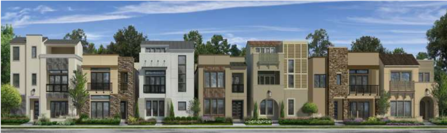
Villas of Legacy West: 126 one, two, and three-story townhomes.
